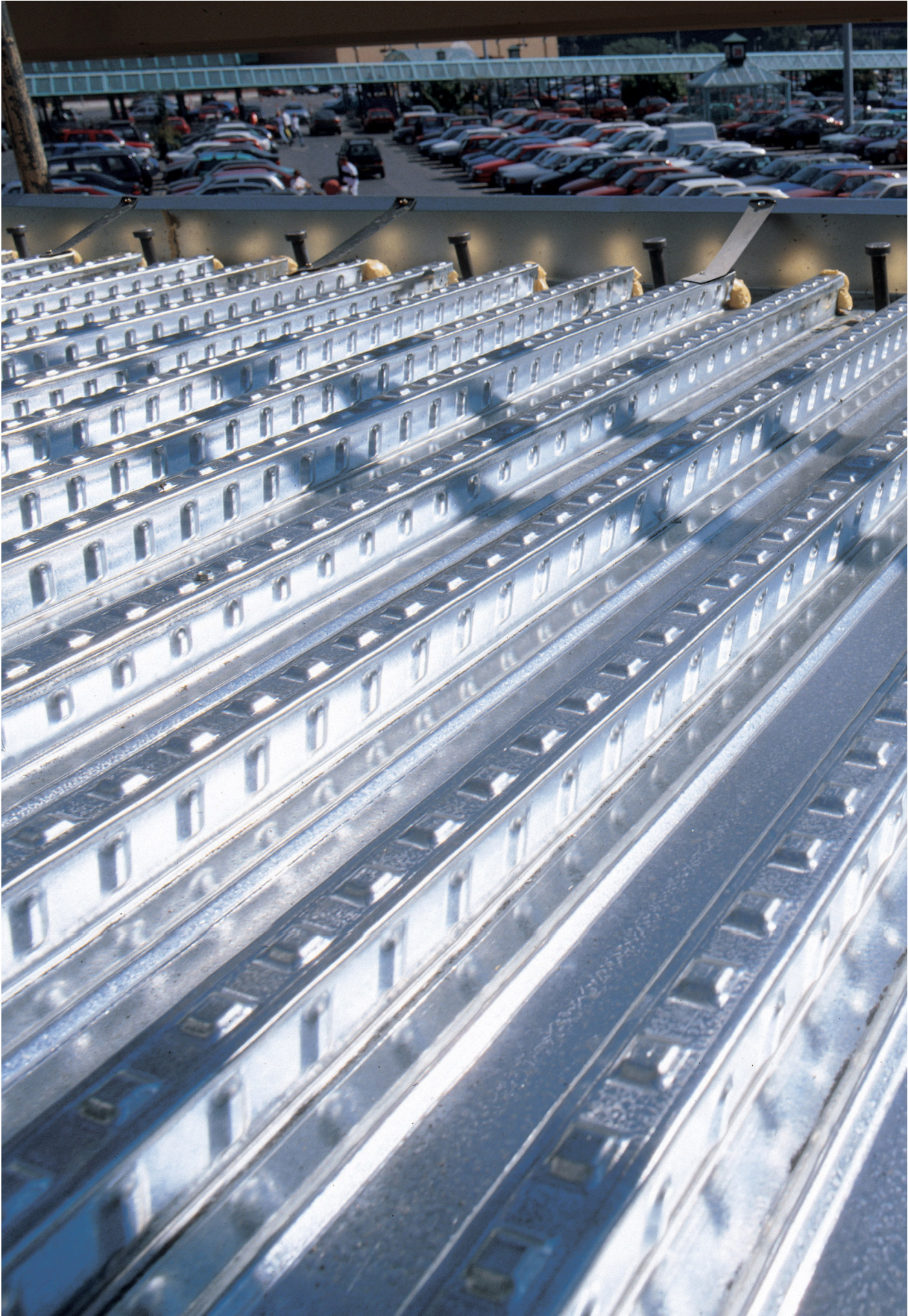
Meadowhall Extension, Sheffield UK. Image courtesy of MSW (UK) Ltd.
